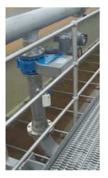
IRIS diaphragm control valve with integrated air/gas flow measuring system ABB Sensyflow.
